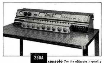
control the 250A Console is the finest unit ever made for AM, FM or TV studio use. Its compactness is made possible by the use of newly designed miniature plug-in preamplifiers, line amplifiers and power supplies. The preamps are only 1 % "x4 $\frac{1}{4}$ "x9". The line amplifiers and power supplies are 2%"x4%"x9". You will find that the new Altec 250A Console leads to better control, more economical operation.
